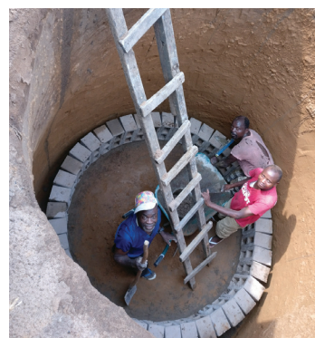
Rehab project - sewer system
